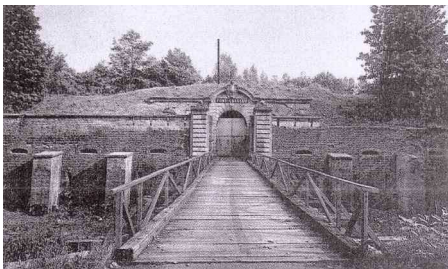
Queuleu Fort entrance. The prisoners were locked in casemate A of the fort. Private collection
